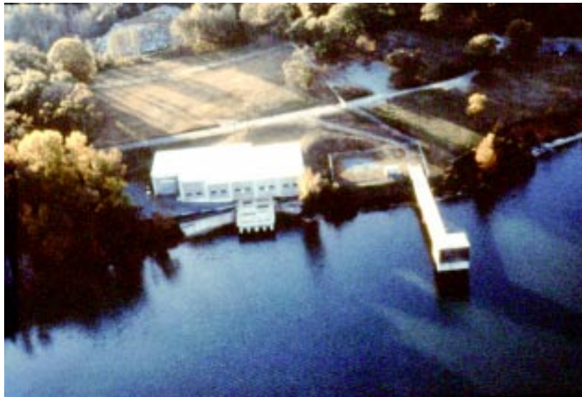
Mount Holly water-supply intake, near Mountain Island Dam (courtesy of Mecklenburg County Department of Environmental Protection)
